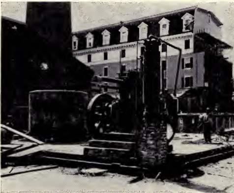
This gasoline engine powered Miami's first electric generator of 40 kilowatts capacity in 1896.
