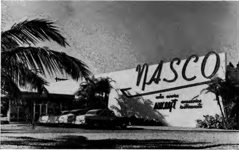
Aviation sparks the sales of aircraft accessories and instruments. This factory faces the Miami airport.
