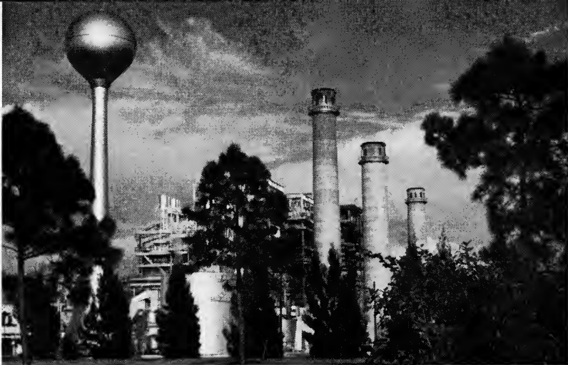
The silver-shining Cutler plant of the Florida Power and Light Company generates 402,000 kilowatts, in 1957.
