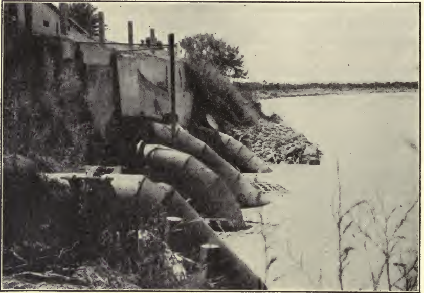
FIG. 97.—The Intake Pipes at the Pumping Station for the Lower Rio Grande Irrigation District (or Division) No. 6, above Brownsville.
