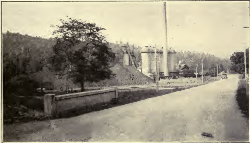
FIG. 118.—The Ferro-phosphate Blast Furnace at Rockdale, in the Nashville Basin. Iron ore and phosphate rock are near at hand. A Nashville Iron worker, J. J. Gray, Jr., after much experimentation, devised a method of making ferro-phosphate in a small blast furnace.
