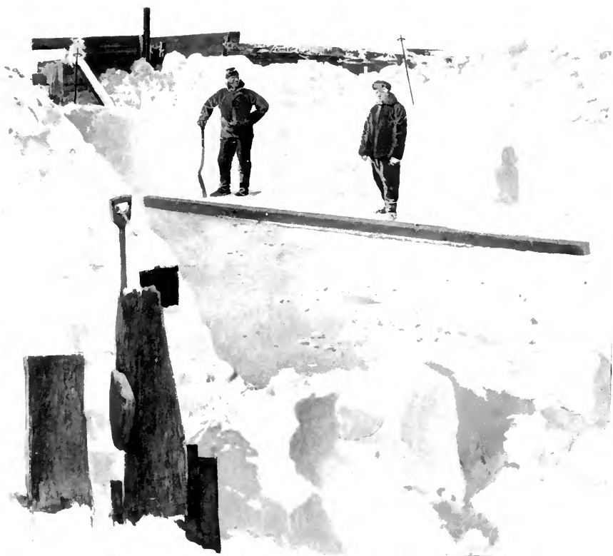
DIGGING THE FOUNDATIONS OF FRAMHEIM.
