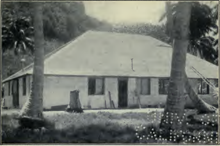
The house nearing completion
