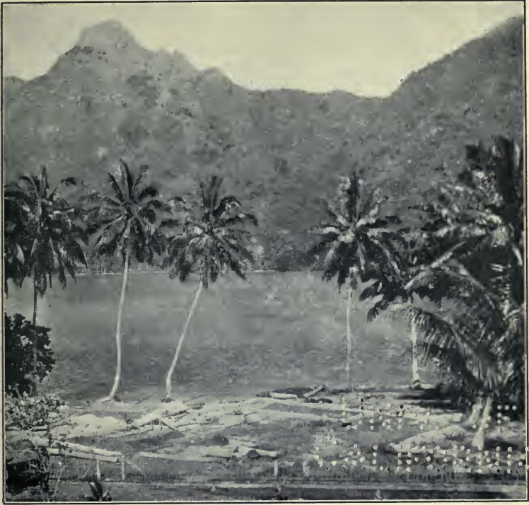
The foundations begun
