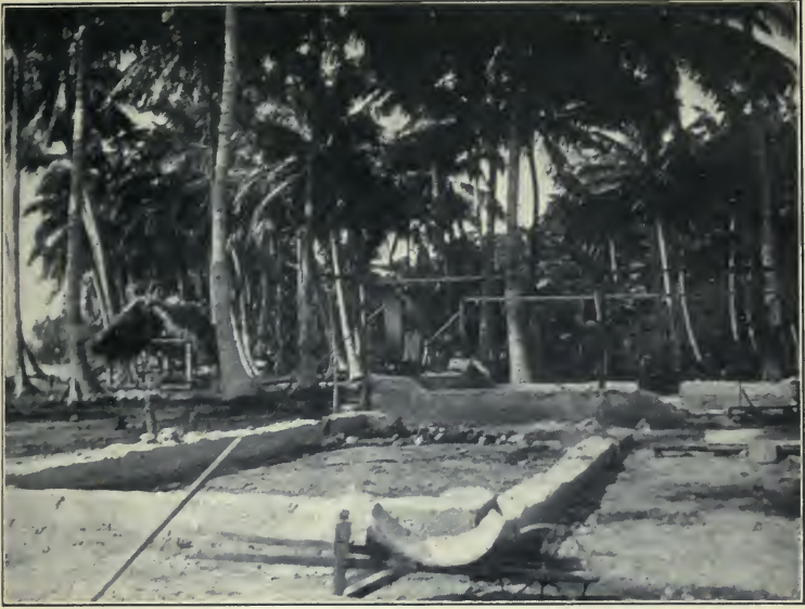
The walls climb up
