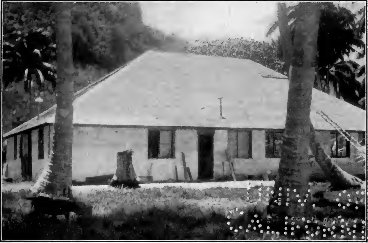
The house nearing completion
