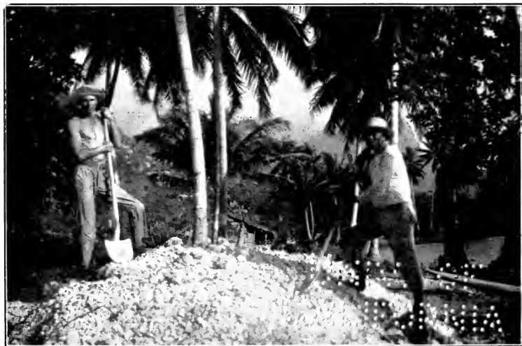
The pit ready to fire
