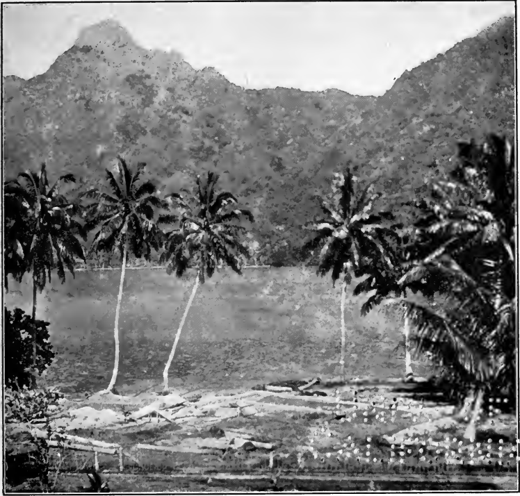
The foundations begun
