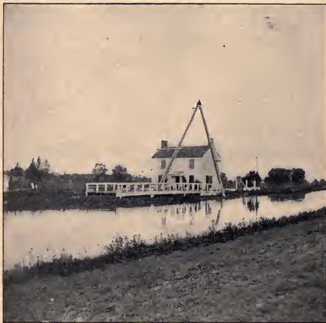
LOCK ON RARITAN AND DELAWARE CANAL
