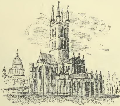
83. SOUTH-EAST VIEW, SHOWING LONDON BRIDGE AND ST. PAUL'S.
