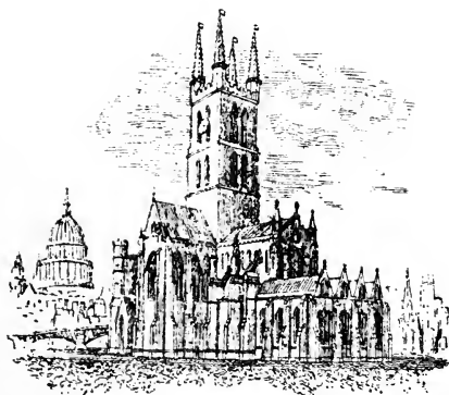
83. SOUTH-EAST VIEW, SHOWING LONDON BRIDGE AND ST. PAUL'S.
