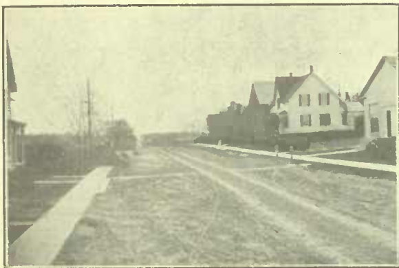
Main Street Looking East
