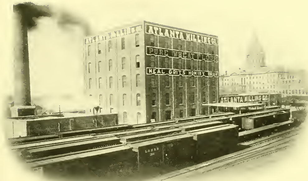
ATLANTA MILLS WITH CAPITOL IN DISTANCE
