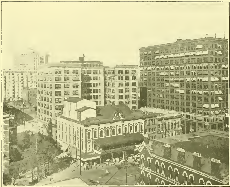
A GROUP OF ATLANTA OFFICE BUILDINGS
