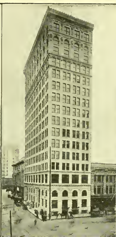
FOURTH NATIONAL BANK BLDG.
