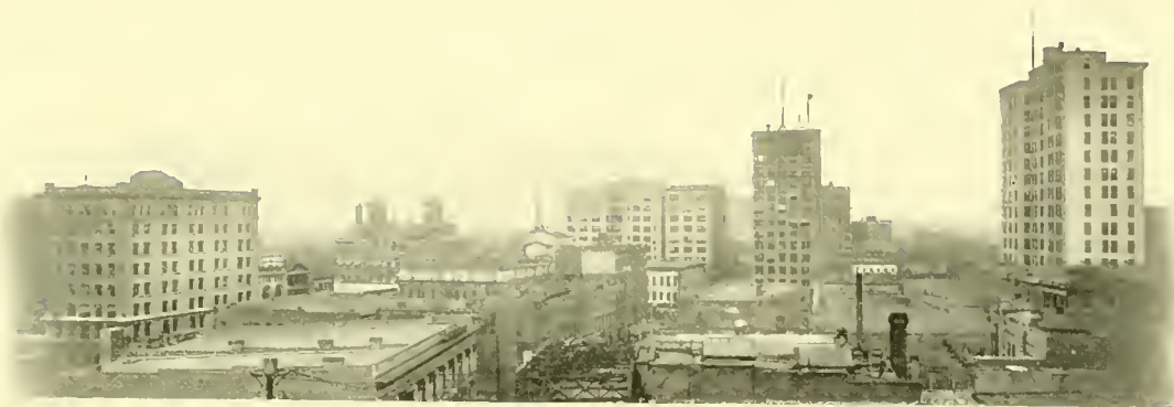
VIEW OF NORTH BROAD STREET
