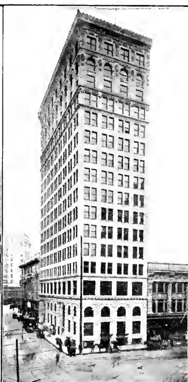
FOURTH NATIONAL BANK BLDG.
