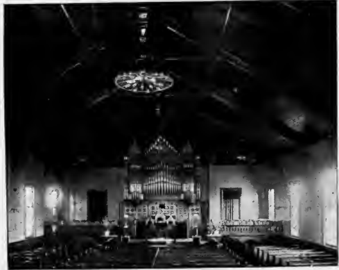
INTERIOR SOUTH MANCHESTER CHURCH.
