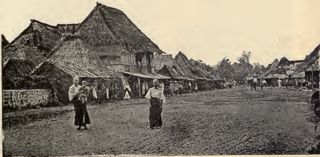
A Native Village. Surrounding Manila are a number of very picturesque native villages. They are constructed entirely of bamboo and thatched with nipa.
