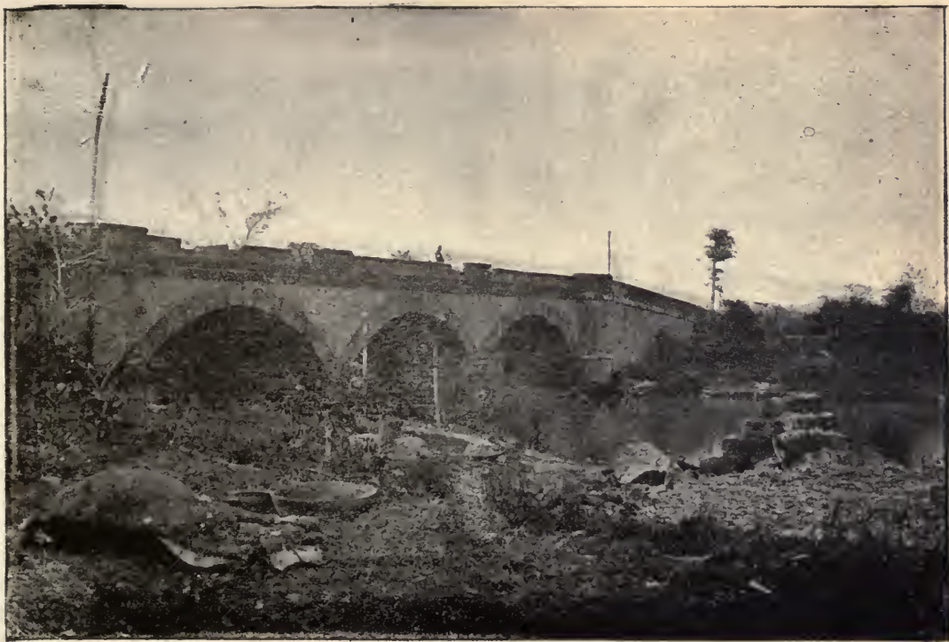
Bridge of San Juan del Monte: This was where the war with the Insurgents started, and where the sons of Nebraska did some hours of hard fighting.
