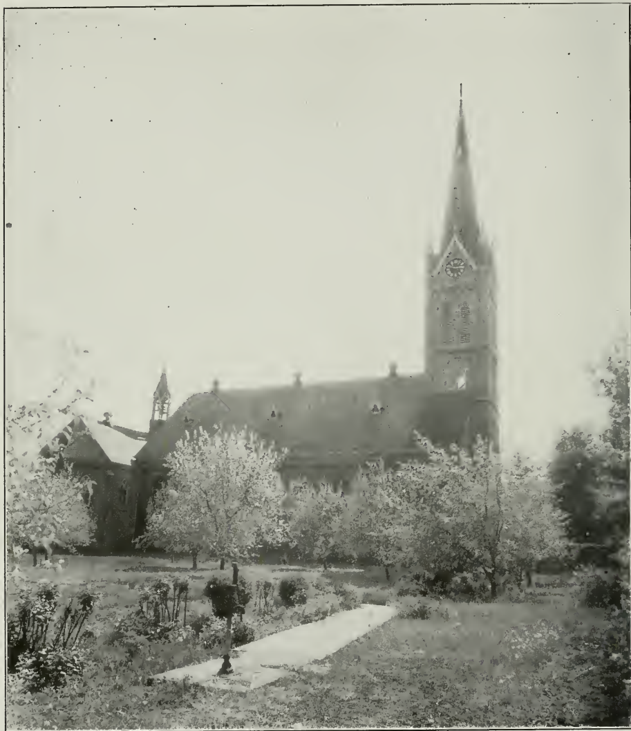
THE PRESENT ST. FRANCIS CHURCH AT TEUTOPOLOIS, ILLINOIS
