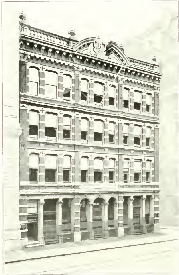
Front View of M. B. Brown Co. Building.
