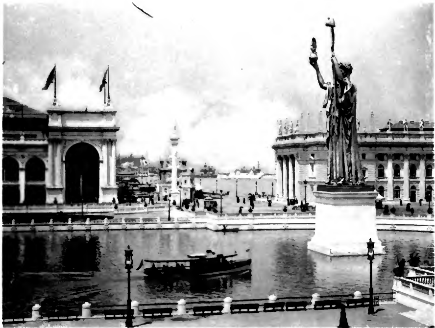
MAIN ENTRANCE OF ELECTRICAL BUILDING AND COURT OF HONOR.
