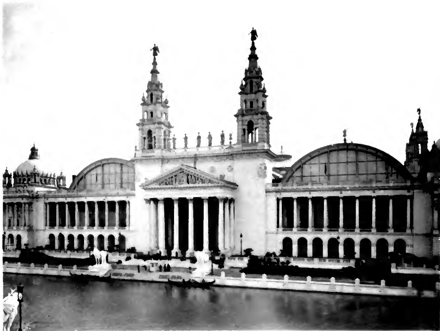
MACHINERY HALL—EAST FRONT.
