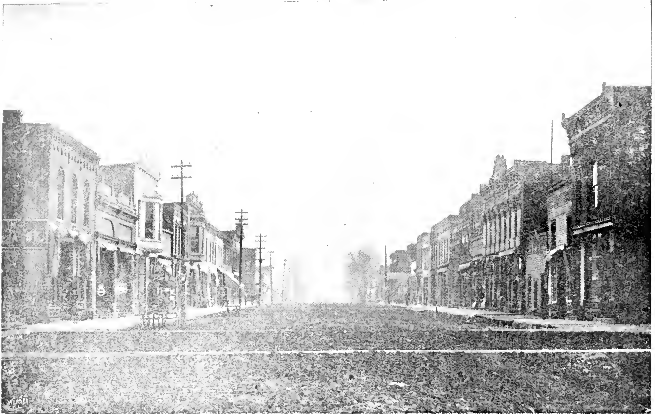
STATE STREET, LOOKING EAST.
