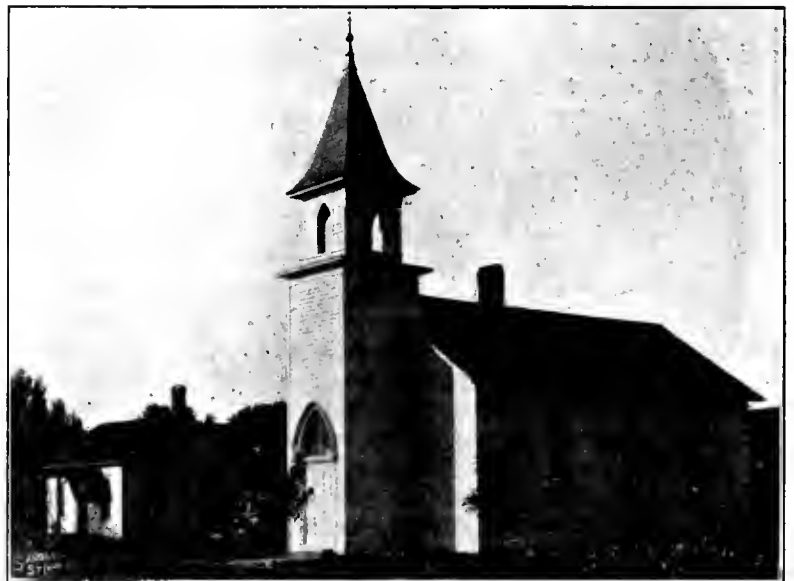
THE GERMAN METHODIST CHURCH AS REMODELED.
