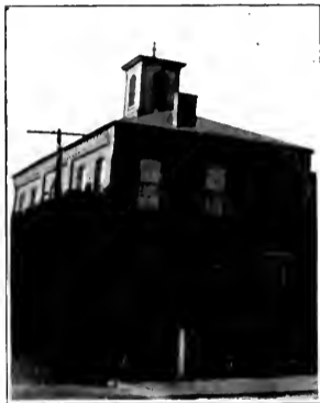
Good Samaritan Hall Cor. 6th and Duvall Streets
