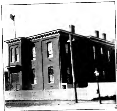
East End School Cor. 29th and O Sts
