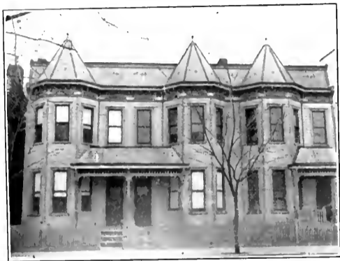
Property of Mr. Jno. O. Lewis 5th Street
