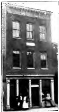
Masonic Hall on Clay Street
