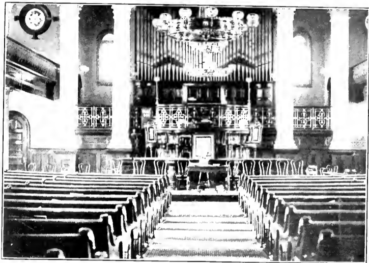
Interior of the First Baptist Church, Rev. W. T. Johnson, Pastor Cor. 14th and Broad Streets (The oldest church in Richmond)
