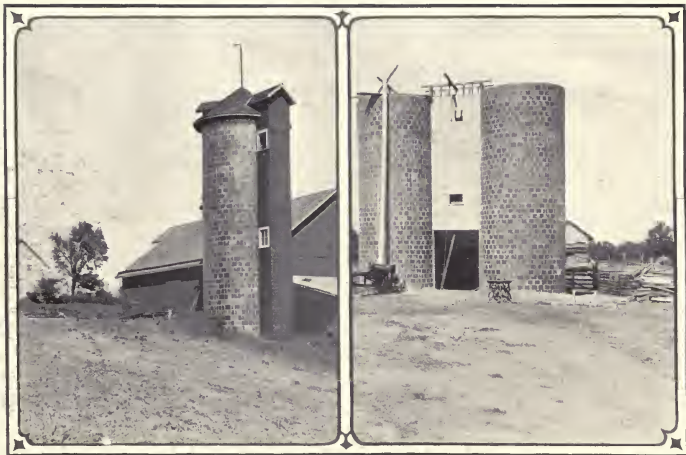
THE GROUT VITRIFIED SILO
