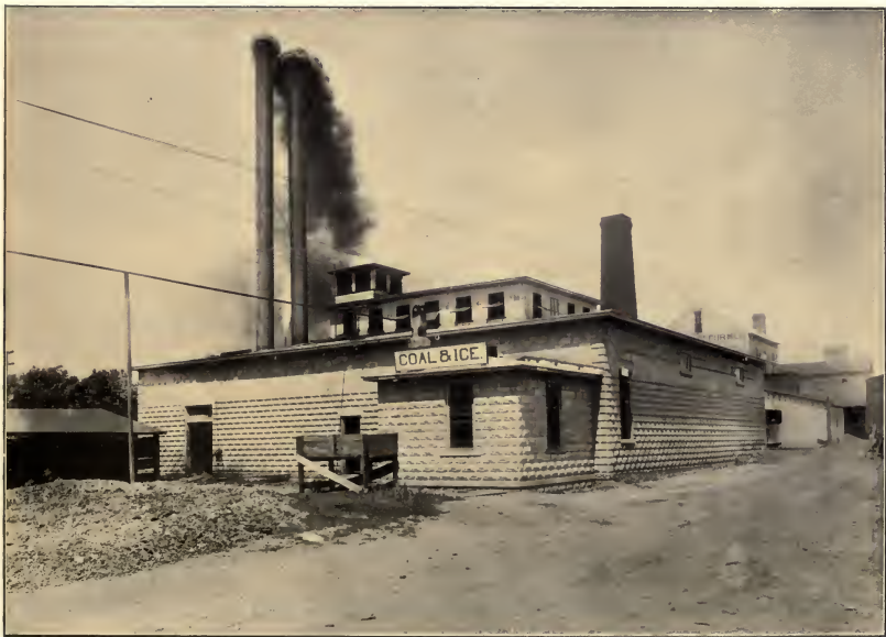
White Hall Ice Company Plant
