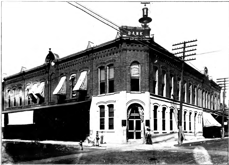
People's Bank Corner
