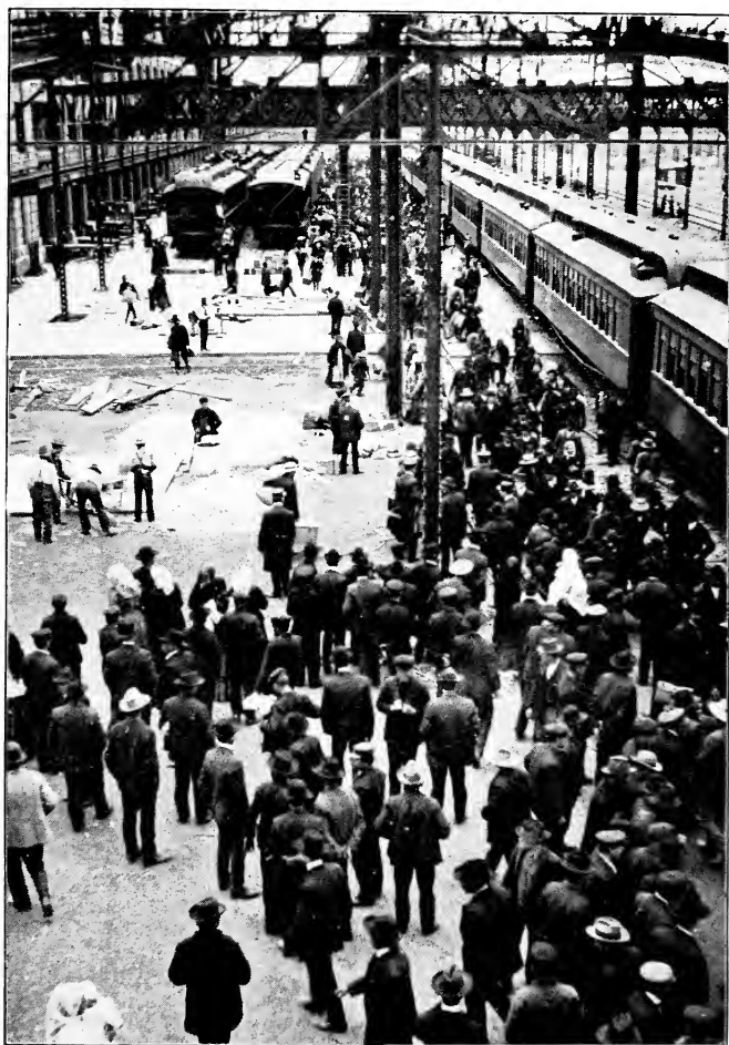
The Royal Alexandra Station at Winnipeg
