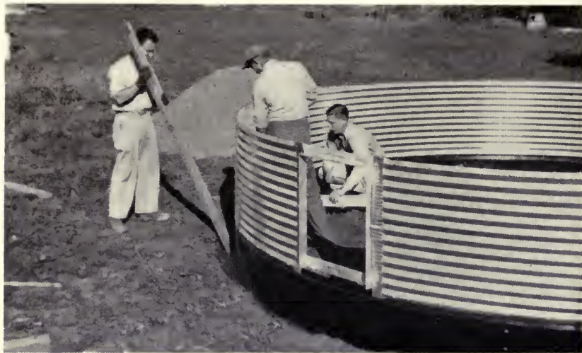
A heavy asphalted metal ring forms the lower portion of the wall and provides a good foundation and excellent anchorage for a metal bin. (Fig. 23)
