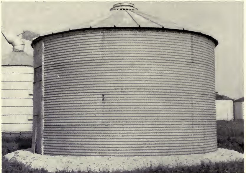
Crushed rock smoothed out, mounded slightly in the center, and extended about 2 feet beyond the wall proved to be a good base for steel-floored steel bins. About 12 cubic yards of rock are needed. (Fig. 22)
