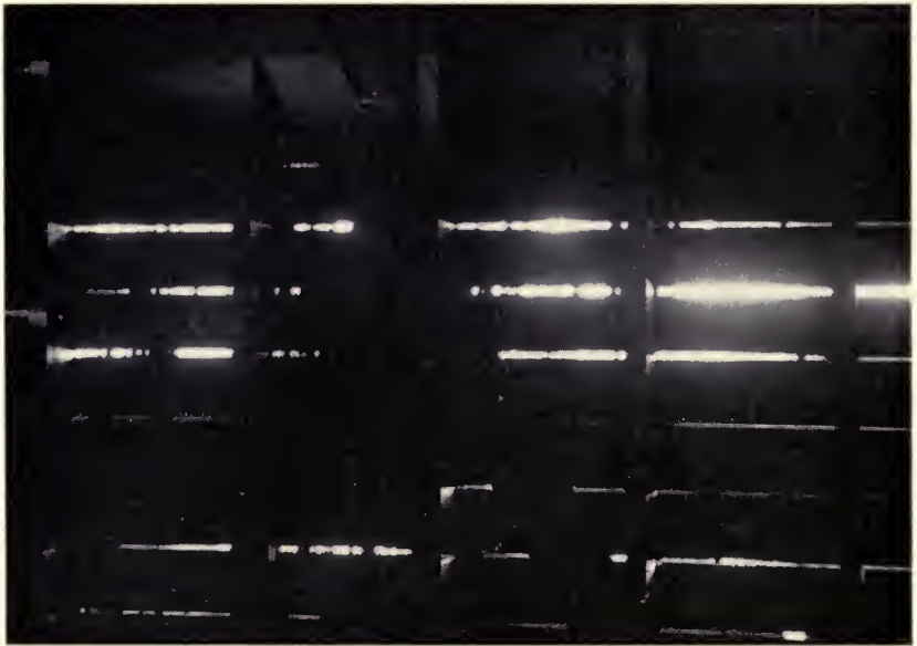
These horizontal cracks resulted from shrinkage of the siding boards. A double covering outside the studding would protect the soybeans. (Fig. 24)
