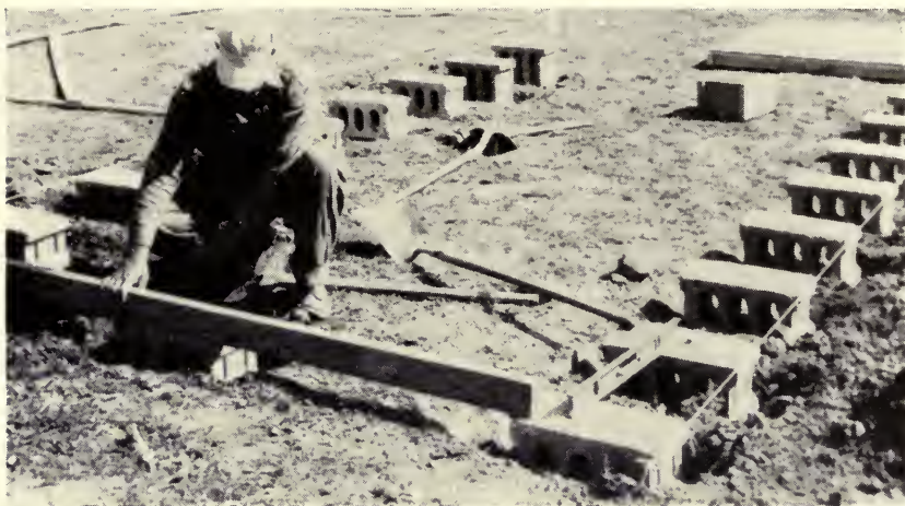
Concrete blocks with the cores horizontal were leveled to make temporary foundations for small bins. (Fig. 19)
