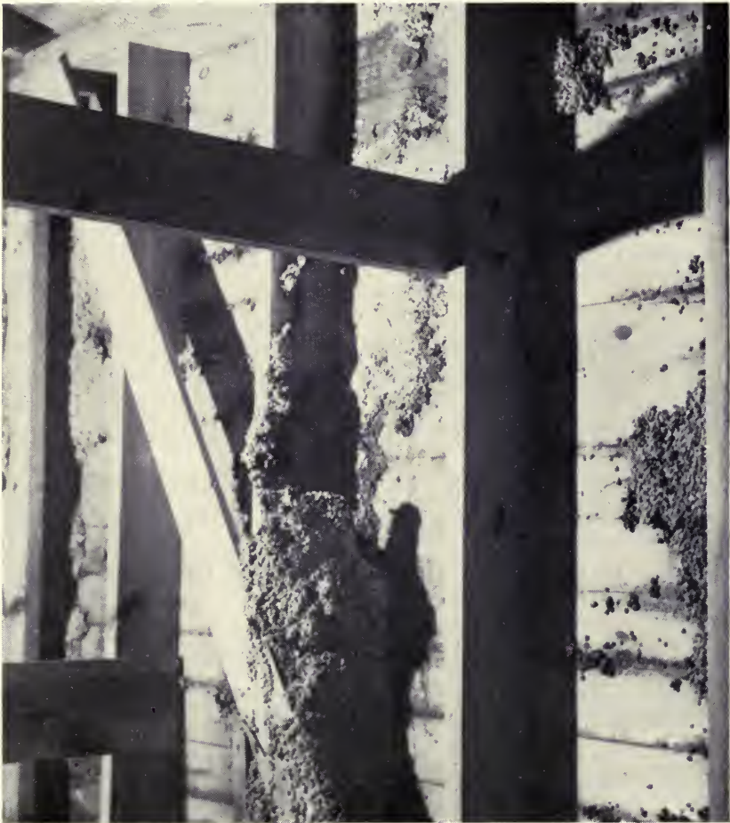
Leaks resulted in damaged soybeans on the inside of bin walls. Reinforced paper lining was not enough to prevent such damage. (Fig. 25)
