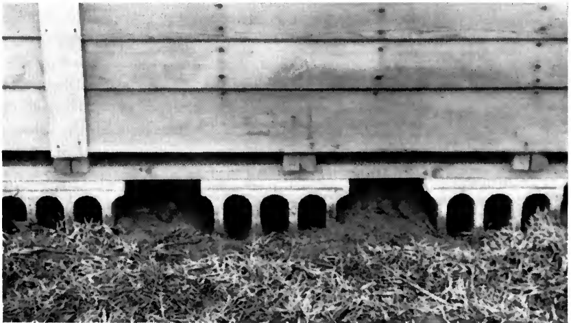
Blocks were placed at right angles with the floor joists under large bins, and a 2-by-6-inch sill was laid across the blocks to keep both the blocks and the joists from tipping. (Fig. 20)
