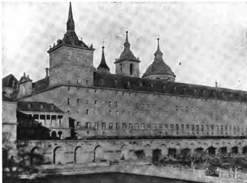
FIG. 136—South Façade of the Real Monasterio de San Lorenzo del Escorial.
