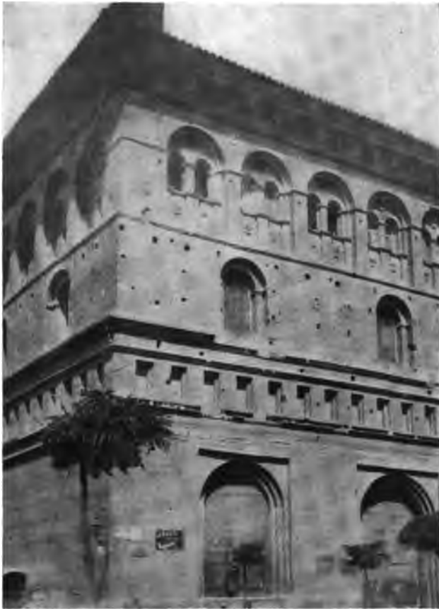
FIG. 112—The Lonja, Zaragoza. Architect unknown. Dated 1551.
