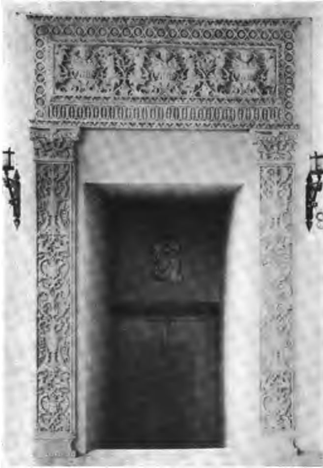
FIG. 82—Doorway in Upper Cloister of the Casa del Duque de Alba, Seville.
