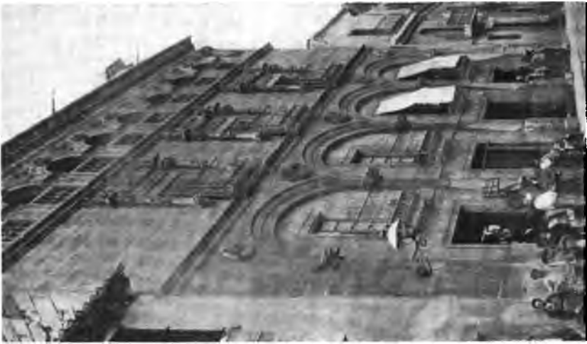
CASA SALINA, SALAMANCA, BEFORE RECENT RESTORATION.
