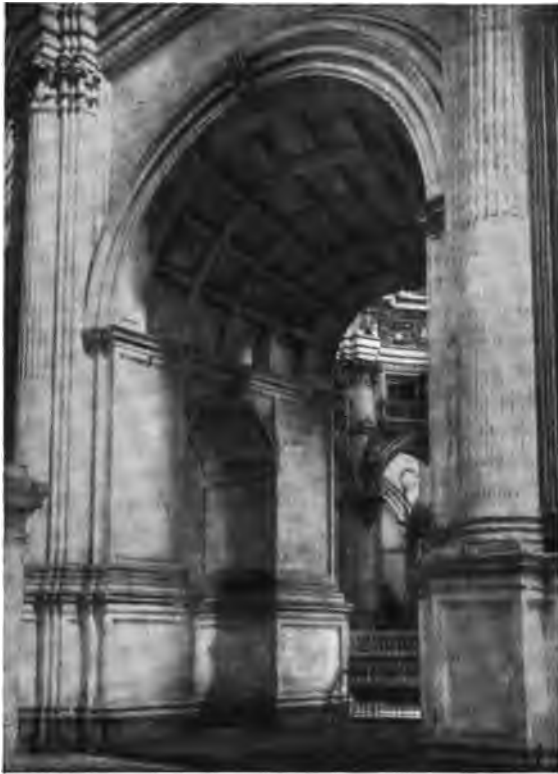
FIG. 89—Ambulatory Arch in Granada Cathedral. Diego de Siloe, Architect, 1525-63.
