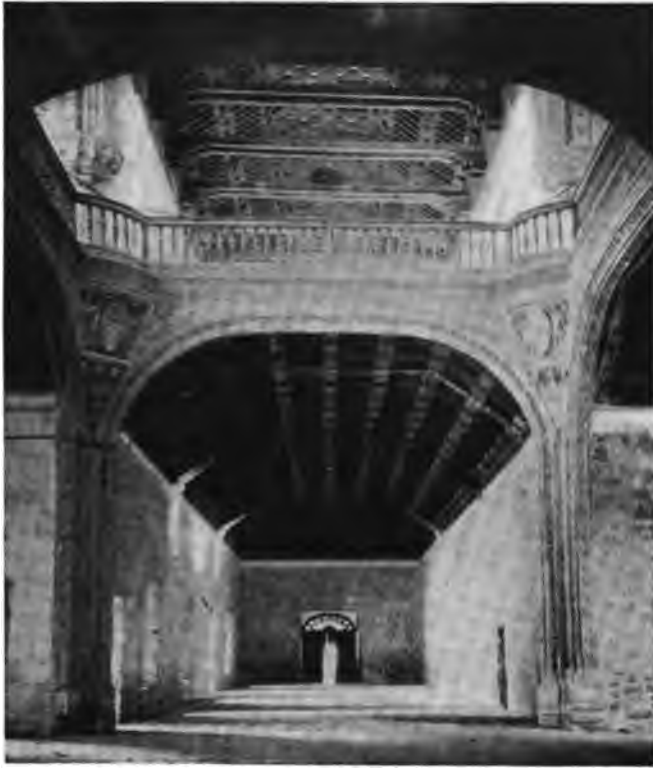
FIG. 5—Interior of the Santa Cruz Hospital, Toledo. Enrique de Egas, Architect, 1504-14.
