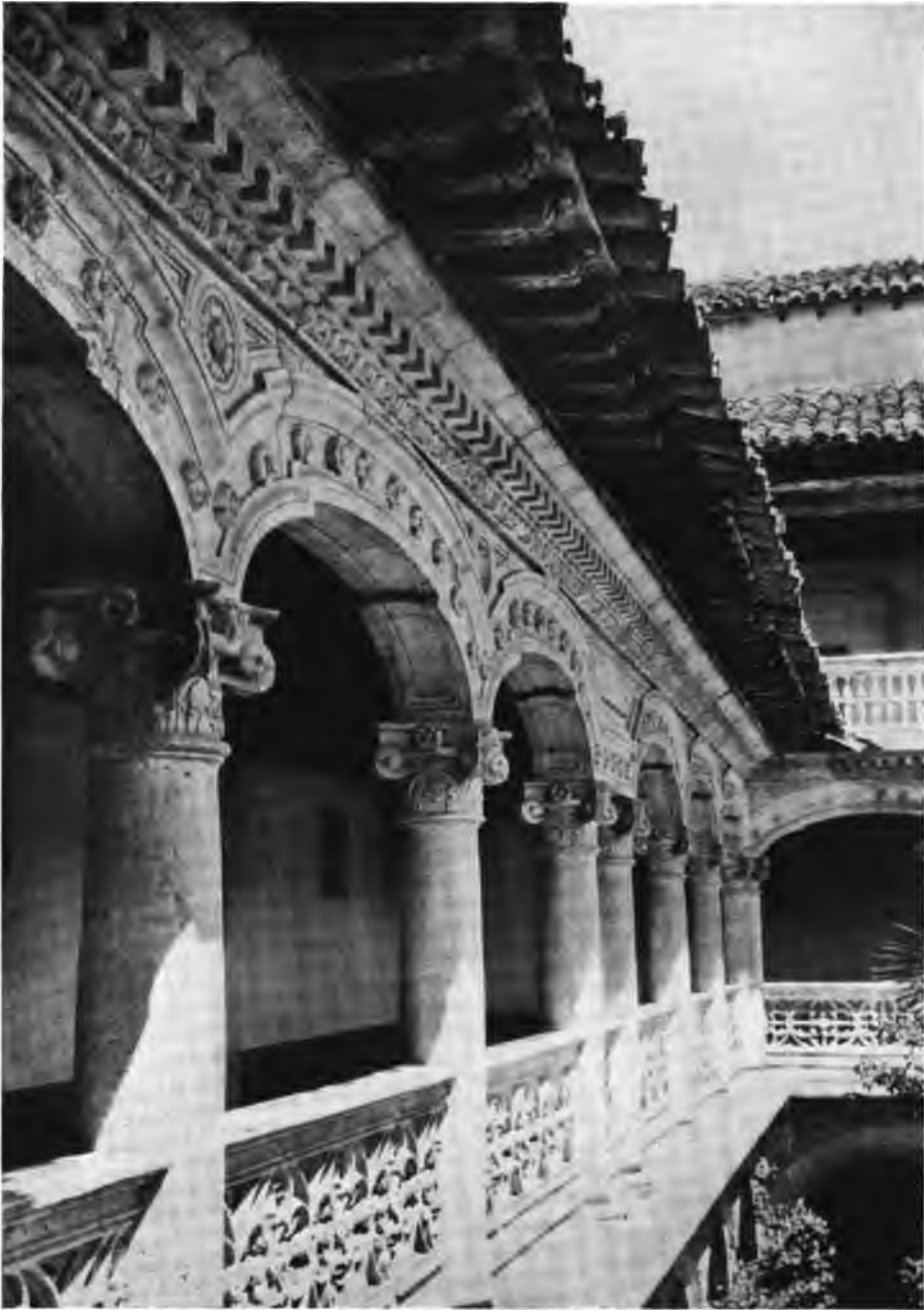
CLOISTER OF THE FORMER HIERONYMITE MONASTERY, LUPIANA.
