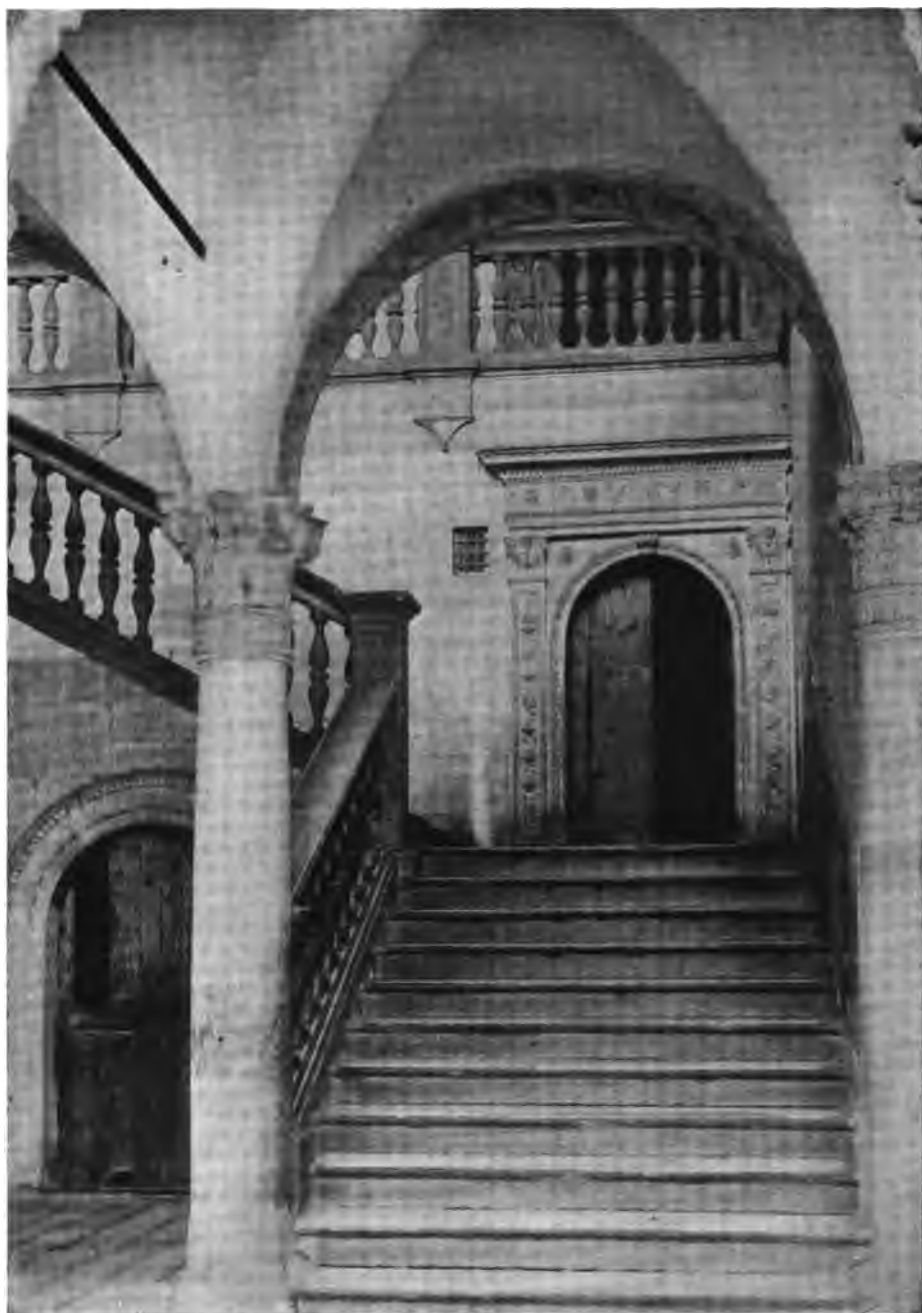
STAIRWAY OF THE CASTILLO DE LACALAHORRA. Michele Carlone of Genoa, Architect, 1508-12.
