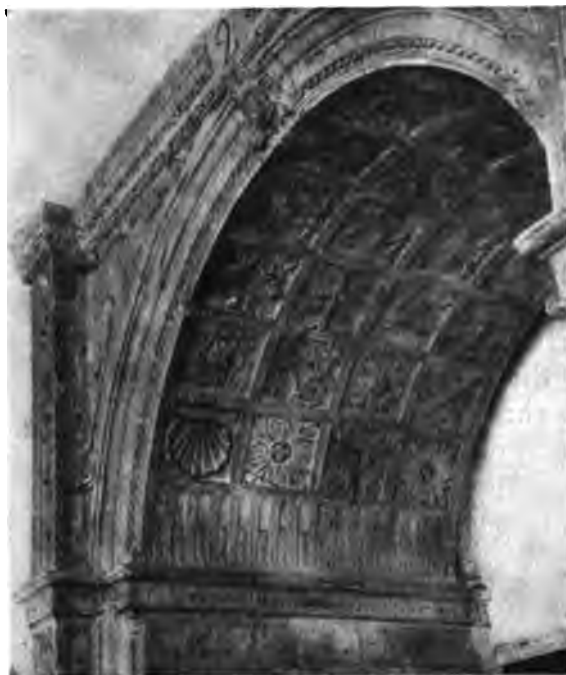
FIG. 29—Detail of an Arch Soffit, Hospital del Rey, Burgos. 1526.
