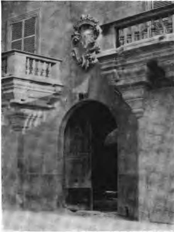
G. 127—Entrance to the Burga-Zaforteza House on the Borne, Palma de Mallorca.
