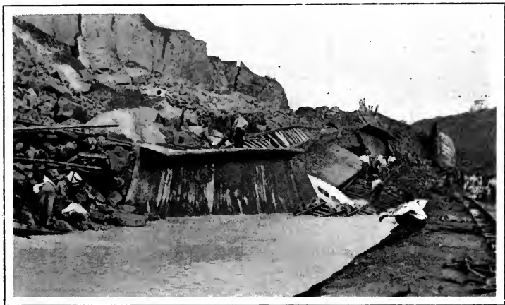
PANAMA CANAL — CULEBRA CUT SLIDE.
