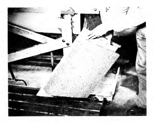
Figure 4.--One of the covers from the experimental tank showing the 3-inch layer of rubberized horsehair used to soundproof the entire inner surface of the tank. In the tank, there was a layer of 1-inch foam rubber under the layer of horsehair.
