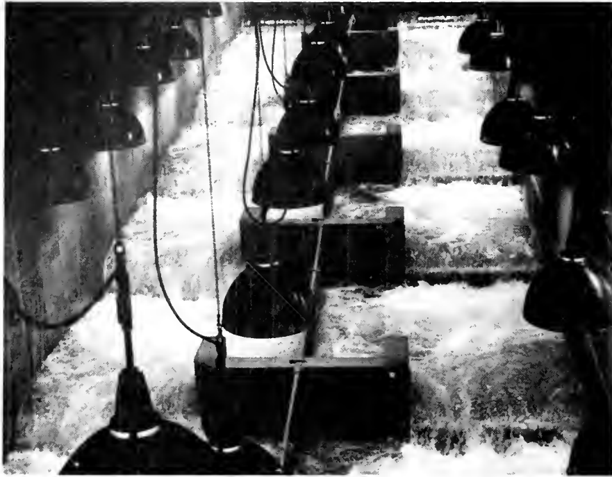
Figure 15.--Operational view of the Ice Harbor fishway with McNary crests on right and The Dalles crests on left. Note reduced turbulence in flow pattern on right. Corners on downstream face of the weir baffles on left are chamfered and those on right squared. Eventual design of prototype was modified to conform with structure on right.
