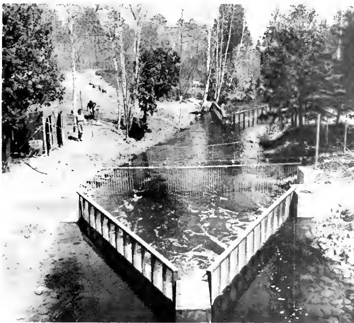
Figure 10. Electrical barrier installed in Carp Creek in 1952 with upper and lower checking weirs.
