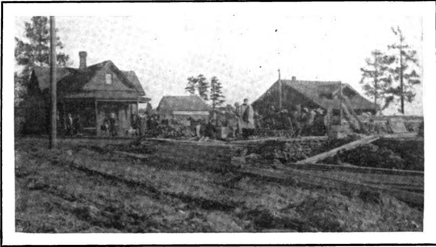
LAYING THE CORNERSTONE OF THE NEW CHURCH OF THE EPIPHANY AT FLAGSTAFF, ARIZONA
