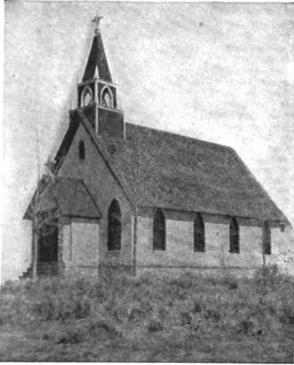
THE CHURCH AT FT. HALL
