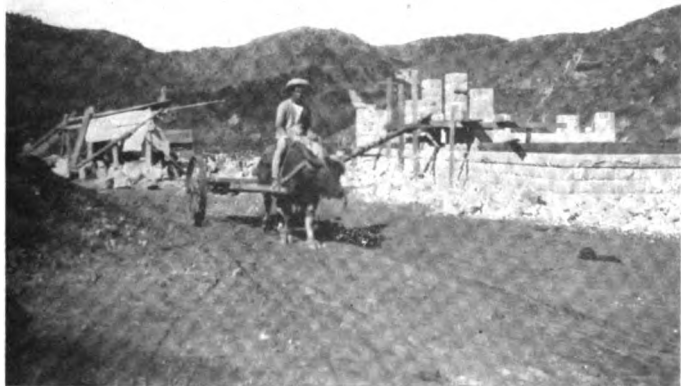
"Do they not build houses of hewn stone?"
