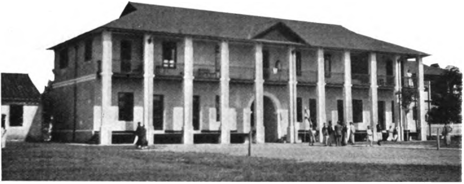
SOOCHOW ACADEMY, MAIN SCHOOL BUILDING
