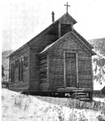
The converted schoolhouse at Placerville
