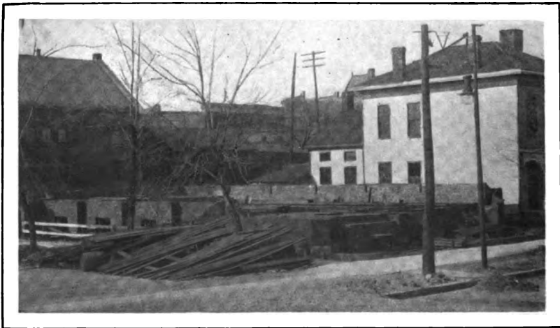
THE FLOOD PUT AN END TO WORK UPON TRINITY CHURCH, PERU, IND.
