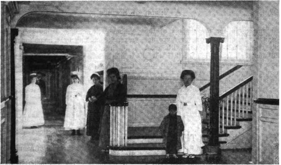
INTERIOR OF THE HOSPITAL
