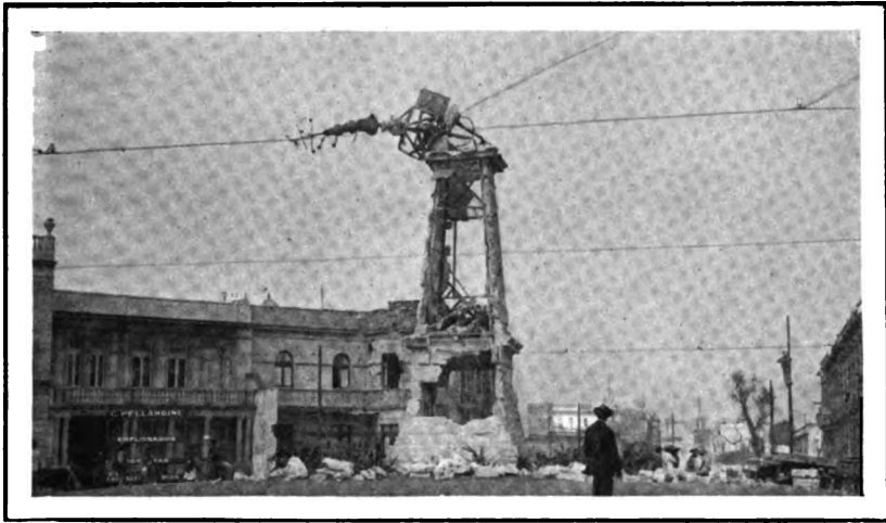
A BADLY DAMAGED CLOCK TOWER CLOSE TO THE HOUSE OCCUPIED BY THE DEACONESSES
