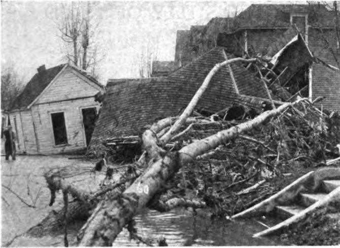
A STREET CORNER IN PERU, IND., AS THE FLOOD SUBSIDED.
