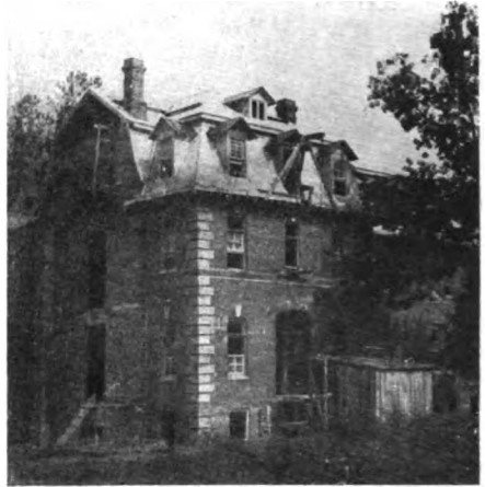
GIRLS' DORMITORY UNDER CONSTRUCTION.
