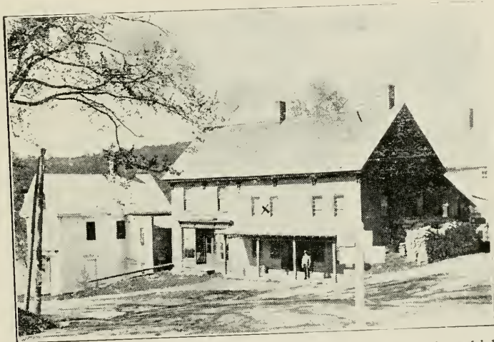
The D. L. Annis building in Sebéc Village, Maine in which was the first law office of Chief Justice Appleton, indicated by X.
