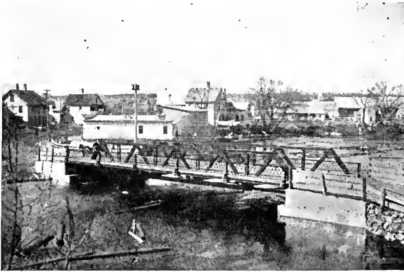
The Moose River Bridge
