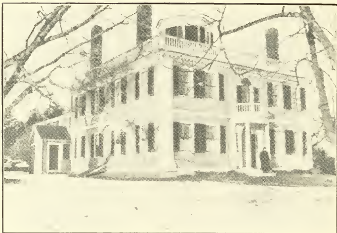
Home of the Hon. Edward Kavanagh, Governor of Maine, 1843, in the village of Damariscotta Mills, town of Newcastle, Maine. For references to Gov. Kavanagh see the Journal (biog. sketch) Vol. II, pp. 37-39, and (in connection with the Northeastern Boundary Controversy) Vol. V, pp. 22-25.
