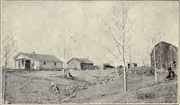
LONG, HARD MONTHS OF WORK SEPARATE THE ROUGH SHANTY FROM WHITE CLAPBOARDS AND AN AUTOMOBILE
