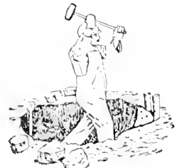
1456. Digging the hole in frozen ground to receive the tree.
