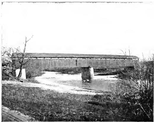
OLD BRIDGES AT BLUFFTON
