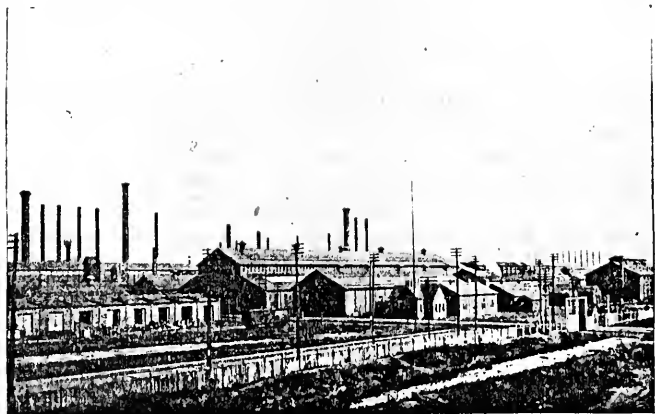
GENERAL VIEW OF SOUTH LORAIN STEEL MILLS
