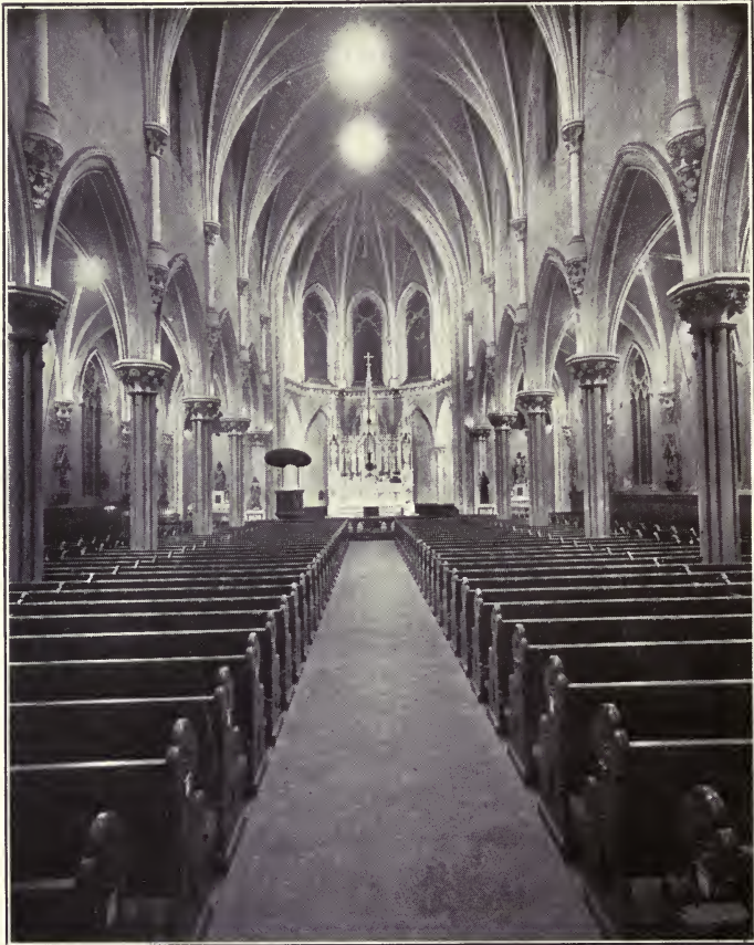
A Combination of Direct and Indirect Illumination is Employed in This Gothic Structure of Light Gray Stone. Deep bowl mirrored reflectors are recessed at the crossings of the arches of the main and side aisles. These are the 300 and 200-watt sizes respectively
