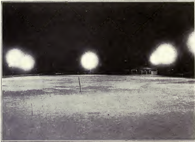
Night View of a Drill Field Lighted by Nine 750-watt MAZDA C Lamps in Angle Steel Reflectors on Poles Around the Edge of the Field
