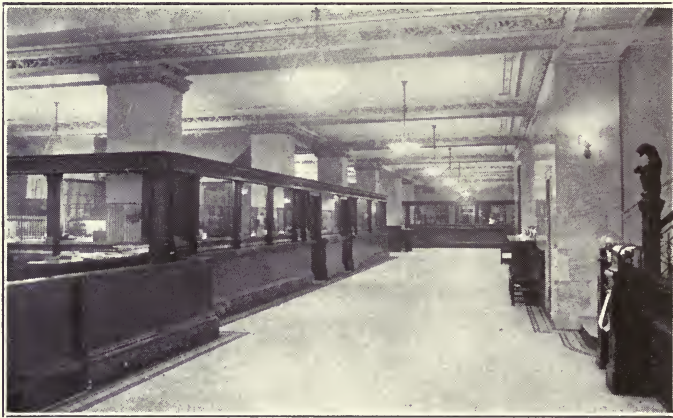
A Well Lighted Bank Using 300-watt MAZDA Lamps in Semi-indirect Bowls on Centers 18 by 32 feet. The fixtures are simple yet dignified and provide a uniform intensity of 5 foot-candles throughout the main banking space
