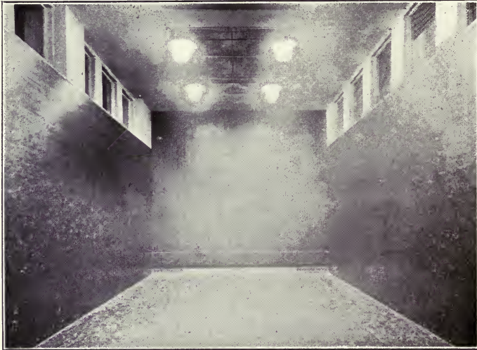
Night View of a Squash Court Lighted by Eight 400-watt MAZDA C Lamps in Opalescent Semi-enclosing Units. The wattage consumption is 5.55 watts per square foot and the intensity is approximately 10 foot-candles
