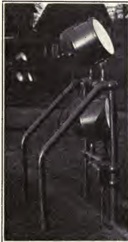
The Wheatena Factory, Rahway, New Jersey—Lighted with 32 500-watt projectors with an average of only 0.41 watts per square foot
