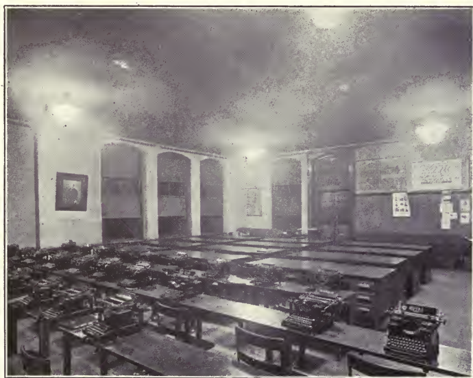
A High Intensity of Illumination if Provided in this Room by 300-watt Clear MAZDA C Lamps in Deep Bowl, Dense Opal, Inverted Reflectors. This type of illumination gives diffusion and eliminates dense shadows
