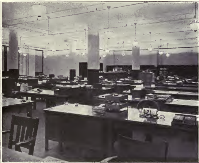
Common Sense Office Lighting of a Modern Type. 150-watt clear MAZDA C lamps are used on 10 ft. centers, 4 outlets per bay. The resultant illumination is slightly over 9 foot-candles
