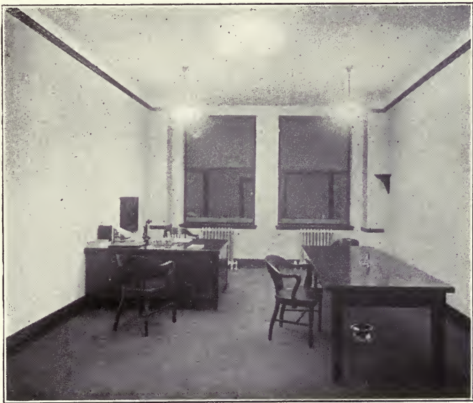
Semi-Indirect Lighting in Small Office
