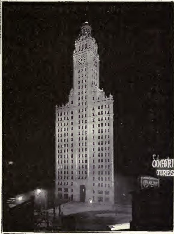
The Wrigley Building, Chicago—An excellent example of floodlighting employing 198 500-watt and 16 250-watt projectors
