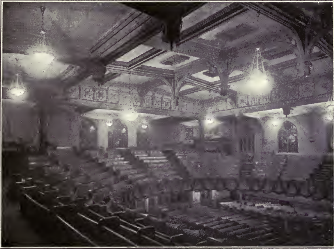
The Smooth Light Colored Ceiling of This Auditorium Lends Itself to the Semi-indirect System. 500-watt MAZDA C lamps are used in the four large central units and eight 200-watt units of similar design are placed above the balcony
