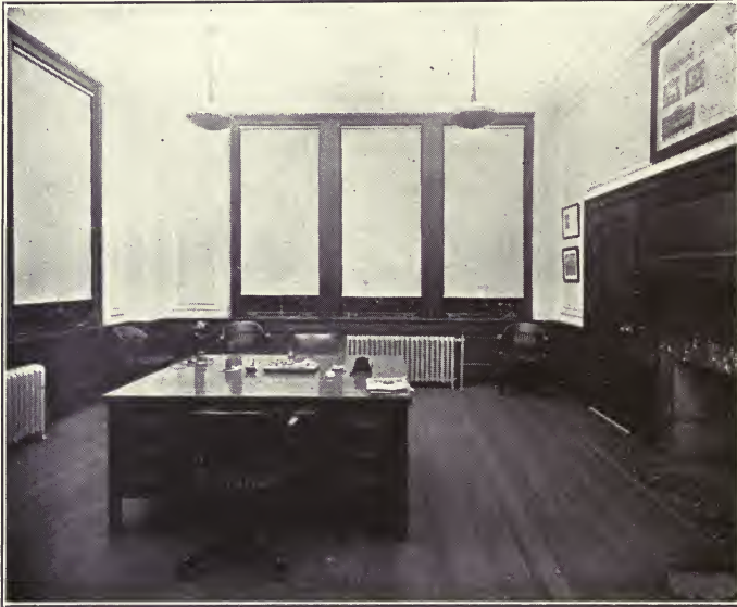
Night View of Totally Indirect Lighting in a Small Private Office. In this installation each outlet supplies 3 75-watt MAZDA C lamps which are placed in inverted mirrored-glass reflectors concealed in a spun metal housing. The intensity of illumination is approximately 9 foot-candles
