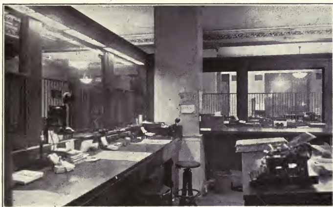
A Night View Showing a Typical Cage Grill Fixture Employing 25-watt MAZDA Lamps Spaced about 14 Inches Apart
