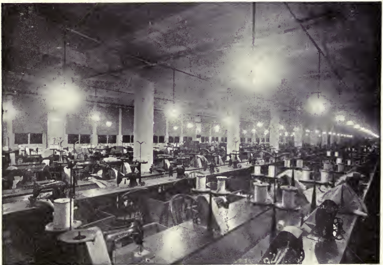
Fig. 14—Shirtwaist factory, sewing machine lighting. Illumination provided by single mantle gas lamps, equipped with prismatic reflectors. Lamps spaced 9 feet apart with a clearance of 5 feet above working plane.
