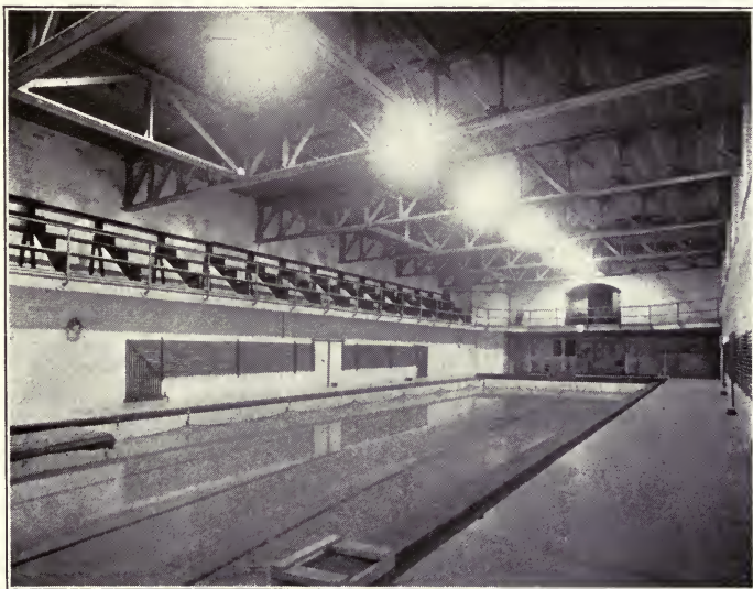
Swimming Pool, 35 x 130 feet, Lighted by 7 200-watt Diffusing Bulb MAZDA C lamps in Dome Enameled Steel Reflectors
