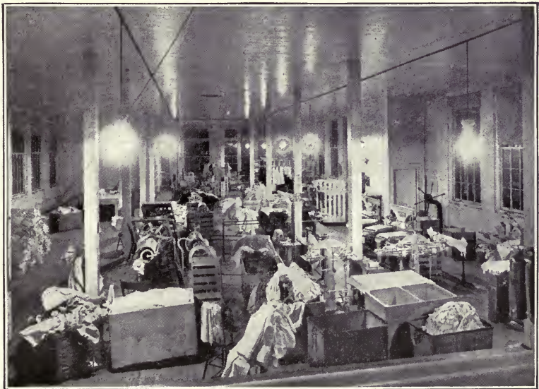
Fig. 16—Laundry lighting—Illumination provided by five mantle gas arc lamps, inclosed type; equipped with diffusing glass globes.
