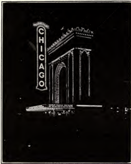
Fig. 6.—Building Outline Lighting with Exposed Lamps
