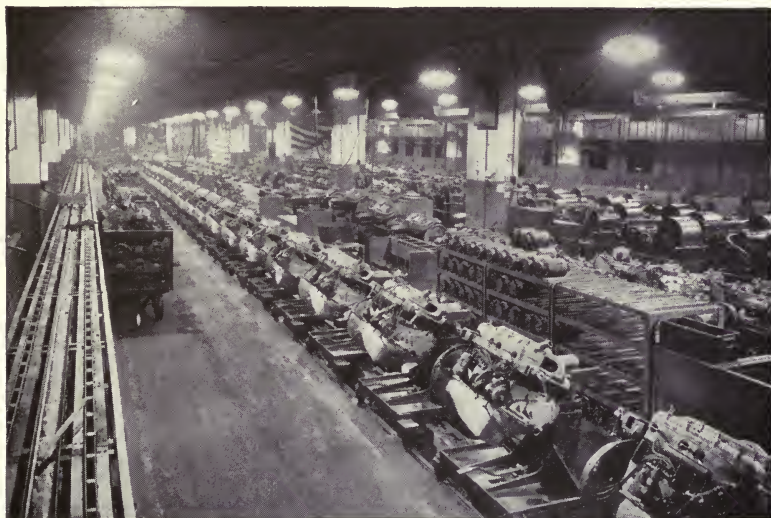
Fig. 4—Freedom from Drop Cords is Essential where Motors are Moving Along in Progressive Assembly
