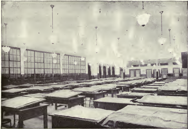
Fig. 11.—Drafting room lighting using dense semi-indirect units and 200-watt lamps. The glazed or shiny ceiling will not increase useful illumination and is frequently a source of glare.
