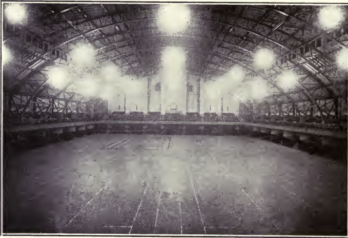
Night View of an Infantry Armory (185 by 275 ft., 40 ft. to Peak) Green Side Walls, Green Ceiling, Light Wood Floor, Lighted by 28 1000-watt Clear MAZDA C Lamps in Two-piece Prismatic Enclosing Units, Steel Cable Suspension
