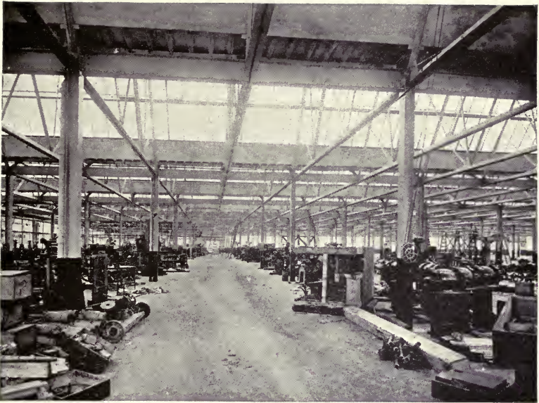
Fig. 1.—Saw-tooth roof construction, with glass facing the north sky, usually results in well diffused daylight illumination.
