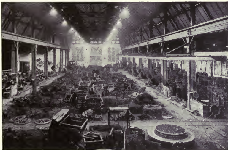
Fig. 3—An Installation of Mirrored-Glass Reflectors in a Foundry
