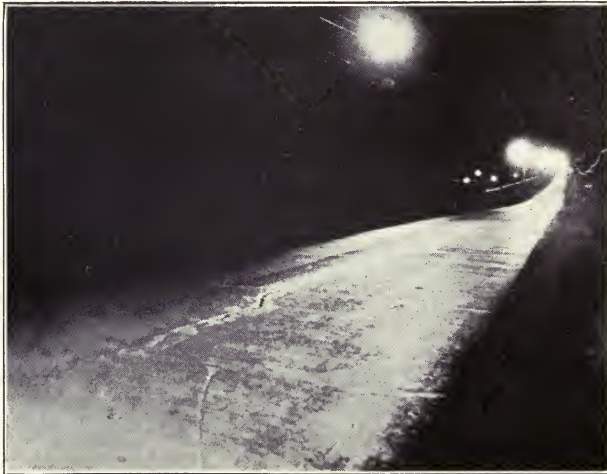
Albany-Schenectady Highway Illuminated by 250 Candlepower Mazda Lamps in Parabolic Units Spaced 300 to 500 Feet Apart and Mounted 30 Feet Above the Ground
