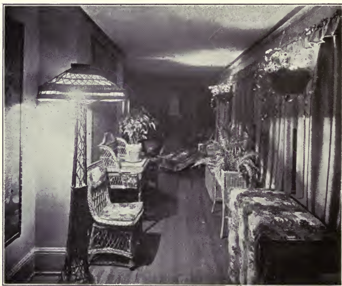
The Indirect Light Sources in This Sunroom Are Inconspicuous by Day and Add to the Decoration When Lighted. 40-watt lamps in metal reflectors are concealed by the artificial flowers in the wire baskets
