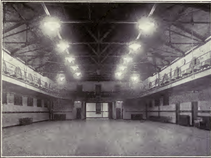
Night Photograph of a Gymnasium 60 by 120 ft., Lighted by 400-watt Clear MAZDA C Lamps in Semi-enclosing Units Consisting of a Diffusing Glass Dish Suspended Beneath a Large Porcelain Enameled Steel Reflector
