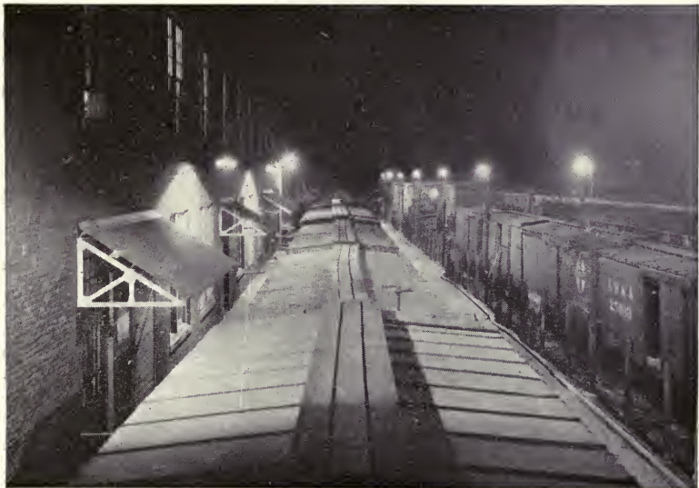
Fig. 12.—A yard lighting installation consisting of 150-watt lamps in shallow bowl reflectors, mounted 20 ft. from the ground. The units in each row are spaced 60 ft. apart, and the two rows are 30 ft. apart.
