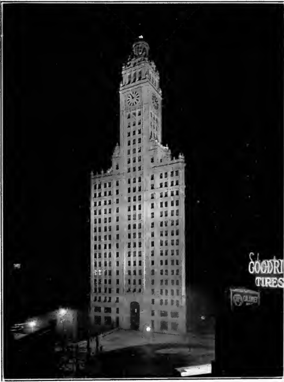
The Wrigley Building, Chicago—An excellent example of floodlighting employing 198 500-watt and 16 250-watt projectors
