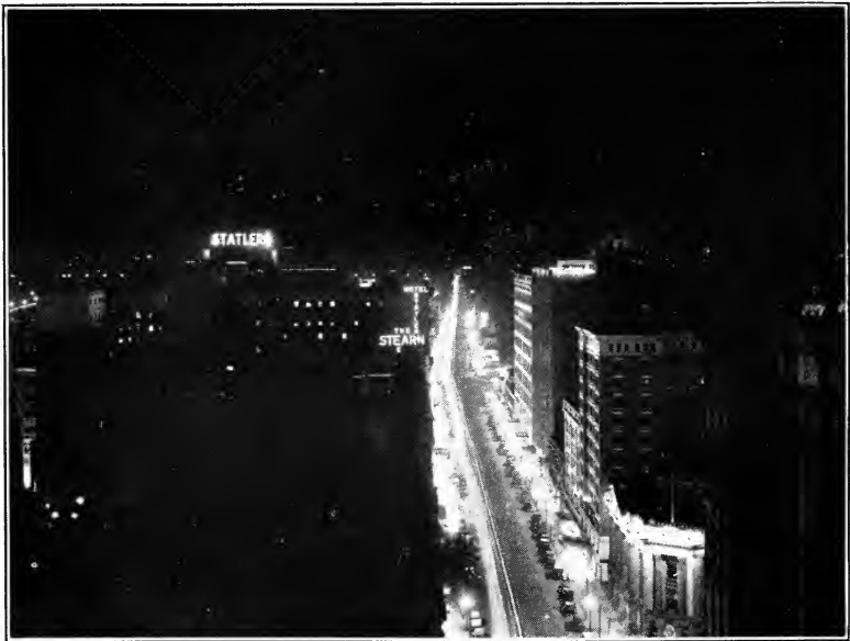
Euclid Avenue, Cleveland, Illuminated by 1500 Candlepower Incandescent Lamps in Ornamental Lanterns Spaced 85 feet apart.
