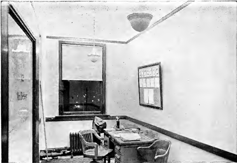
Fig. 10—Lighting an office by means of indirect units. Illumination approximately 6 foot-candles.
