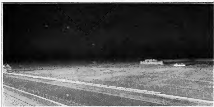
Night View of Sheepshead Bay Speedway Taken from End of Grandstand. The Illumination of the Track and Field is accomplished by MAZDA C Flood-lighting Lamps in Form L-1 Projectors
