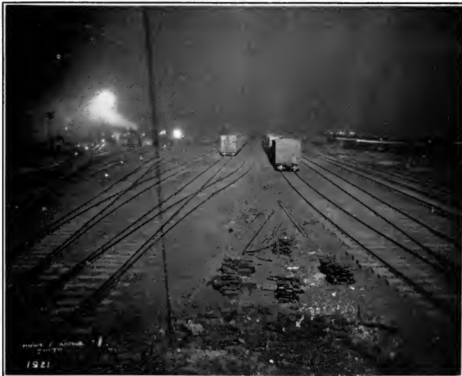
Pennsylvania Freight Yards, Chicago—Lighted by two banks of eight 1000-watt floodlighting units, mounted on towers 75 feet above the tracks. The two towers on which they are mounted are 3000 feet apart with beams opposed
