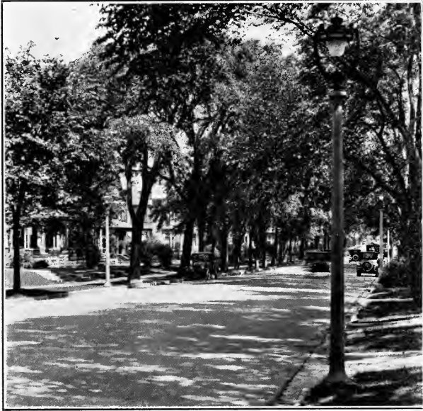
Prospect Avenue, Milwaukee, Wis. 15 foot concrete posts, 120 feet apart, 42 lumens per lineal foot of street. Average intensity, 0.2 foot candles
