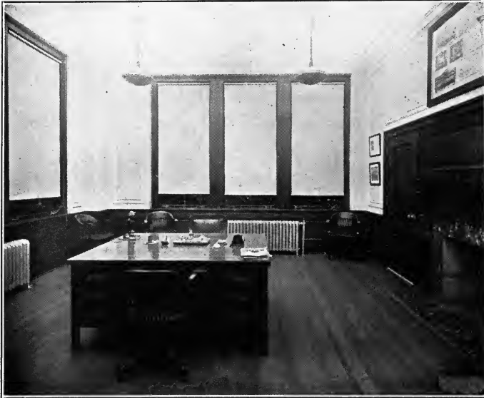
Night View of Totally Indirect Lighting in a Small Private Office. In this installation each outlet supplies 3 75-watt MAZDA C lamps which are placed in inverted mirrored-glass reflectors concealed in a spun metal housing. The intensity of illumination is approximately 9 foot-candles
