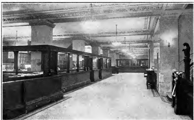
A Well Lighted Bank Using 300-watt MAZDA Lamps in Semi-indirect Bowls on Centers 18 by 32 feet. The fixtures are simple yet dignified and provide a uniform intensity of 5 foot-candles throughout the main banking space
