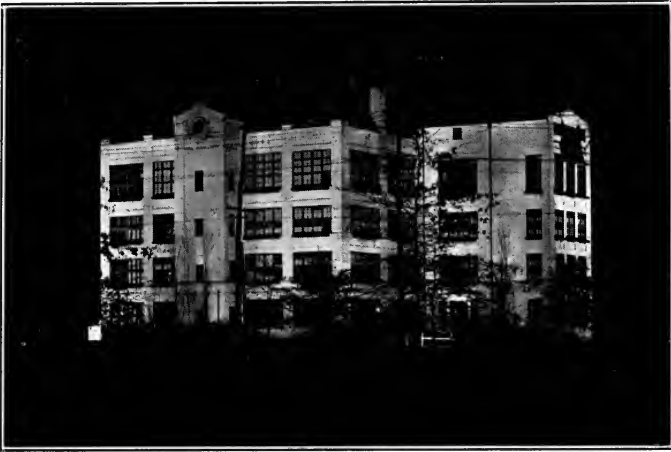
The Wheatena Factory, Rahway, New Jersey—Lighted with 32 500-watt projectors with an average of only 0.41 watts per square foot
