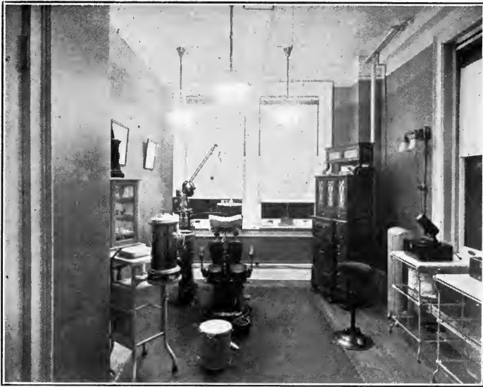
A Small Dental Office Lighted by Three 200-Watt MAZDA Daylight Lamps in Simple Type Semi-indirect Bowls. A uniformly distributed high intensity illumination of suitable color is produced. The diffused character of the light is particularly valuable for illuminating the recesses of the mouth
