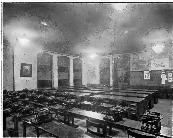
A High Intensity of Illumination if Provided in this Room by 300-watt Clear MAZDA C Lamps in Deep Bowl, Dense Opal, Inverted Reflectors. This type of illumination gives diffusion and eliminates dense shadows
