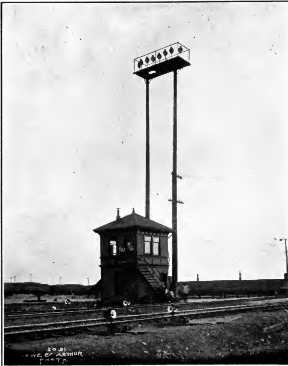
Pennsylvania Freight Yards, Chicago—Two-pole tower mounting eight 1000-watt Floodlight Units. Two such towers are employed 3000 feet apart, with beams opposed.
