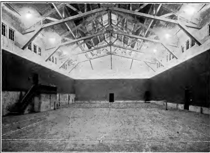
Night View of a Tennis Court Showing Lighting Effects Obtainable with a Combination of Semi-indirect and Totally Indirect Lighting. Eight 750-watt MAZDA C lamps are used
