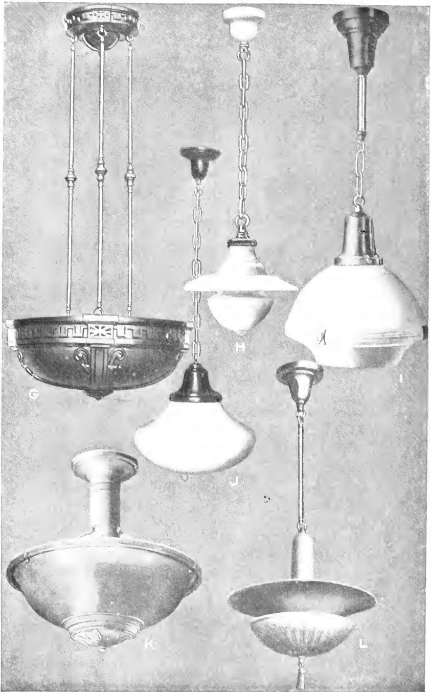
Fig. No. 1A—Typical Store Lighting Luminaires
