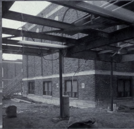
Looking into what will be the new gallery.
