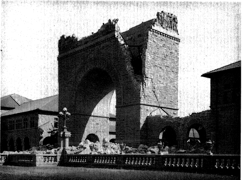
Memorial Arch after the earthquake
