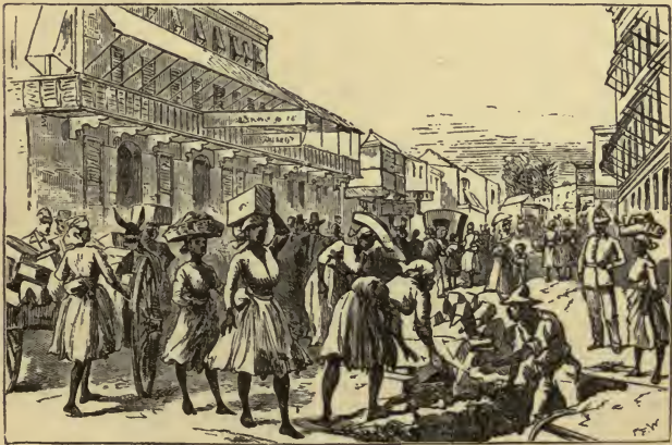
REPAIRING THE ROAD.
