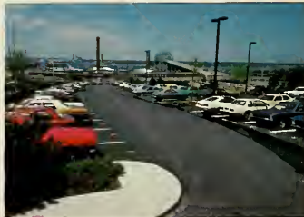
Top Photo: For the Seekonk, Massachusetts location of Ann & Hope stores, full site and civil services were provided for the ingress/egress, parking, lighting and landscaping in conjunction with store design.
