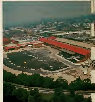
Arsenal Marketplace, the $45 million conversion/renovation of the Watertown Arsenal, was totally site engineered by LEA with additional responsibilities for the adjoining municipal street reconstruction.
