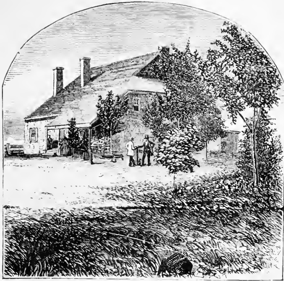
WASHINGTON'S HEADQUARTERS AT NEWBURG.
