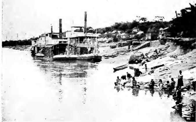
PORT ON THE MAGDALENA AT GIRADOT, COLOMBIA
