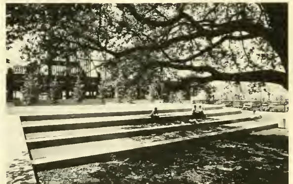
Adjacent to the two specimen live oaks preserved on the site are large circular retaining walls that terminate the grassy mound and provide space for informal sitting.
