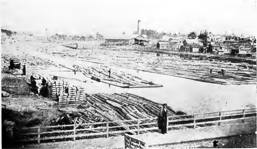
BLACK RIVER, LOOKING WEST FROM MILITARY STREET BRIDGE. 1863
