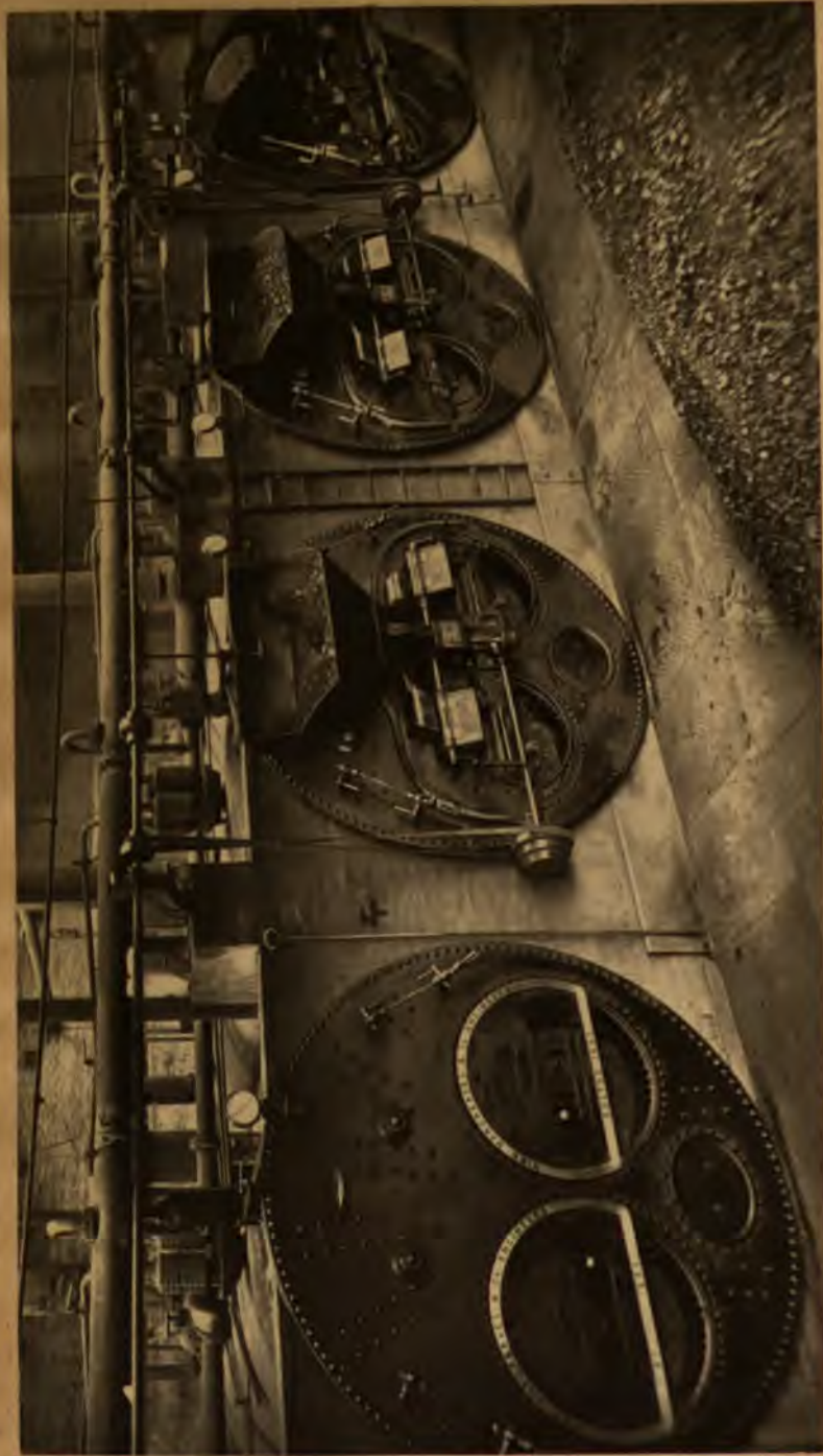
RANGE OF LANCASHIRE BOILERS BY HICK, HARGREAVES & CO., BOLTON.
