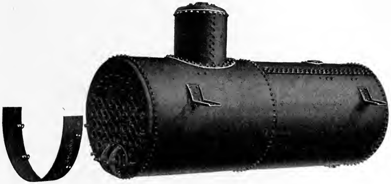
FIG. 4.—Horizontal fire-tube boiler with dome.
