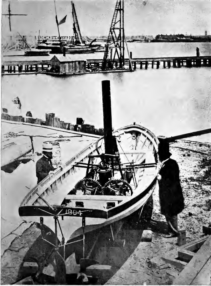
STEVENS' 1804 ENGINE, FITTED INTO OPEN BOAT WITH TWIN-SCREW PROPELLERS
