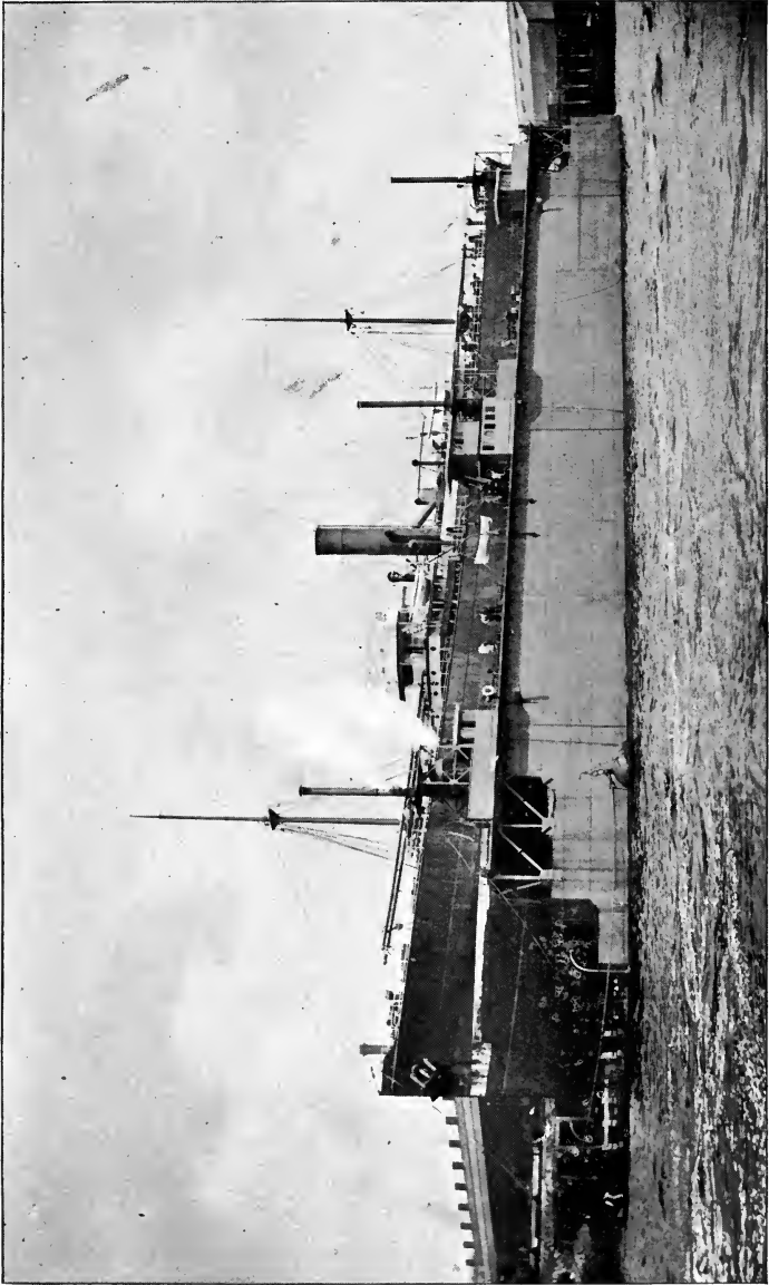
BOLTED SECTIONAL DOCK LIFTING A VESSEL.
